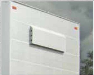
Vent with Rain Deflector
