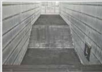
Graphite Applied to the Floor
