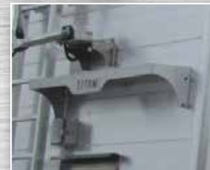
Front and Rear Catwalks
